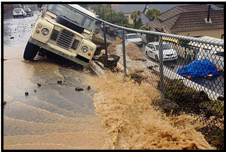
Canterbury Street Retaining Wall. Image: Treesa Green
