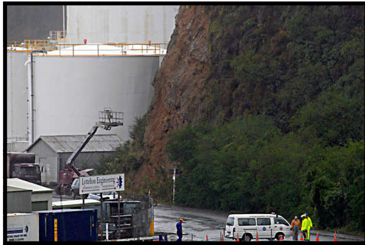
Cliff Collapse onto Tank Farm. Image: The Press | Daniel Tobin
