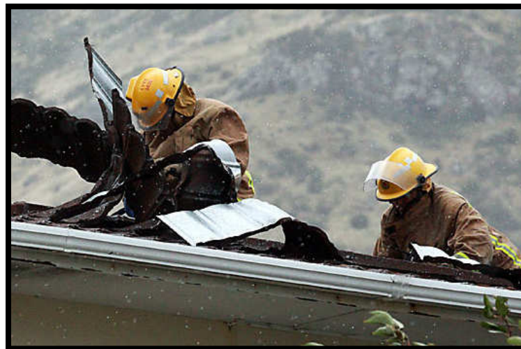
Cass Bay Roof Lifting. Image: The Press | Stacy Squires
