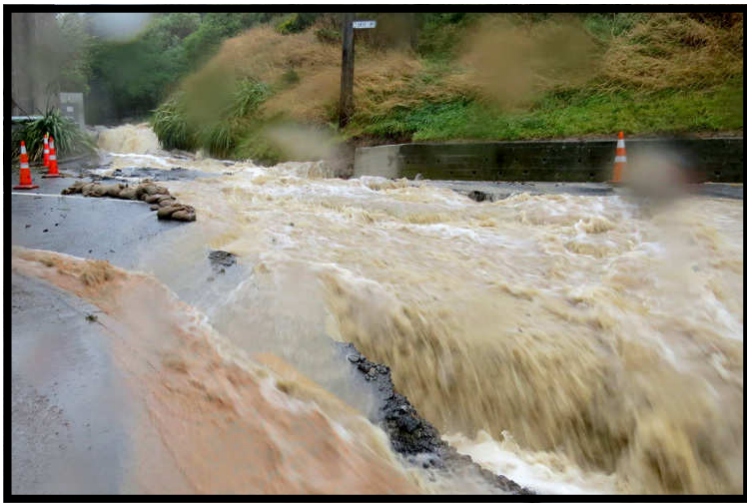
Canterbury Street Junction with Days Road. Image: Bryan Shankland
