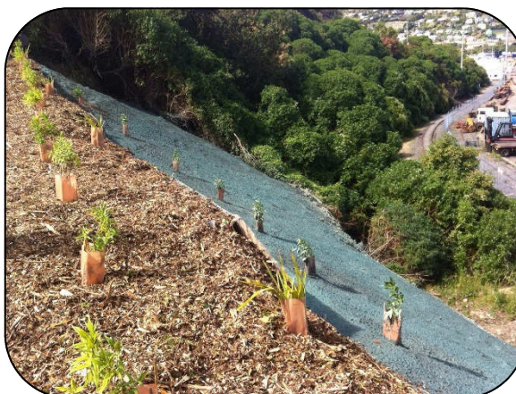
The slope has been planted and hydroseeded. The seed appears as a green mat until the seed germinates.
