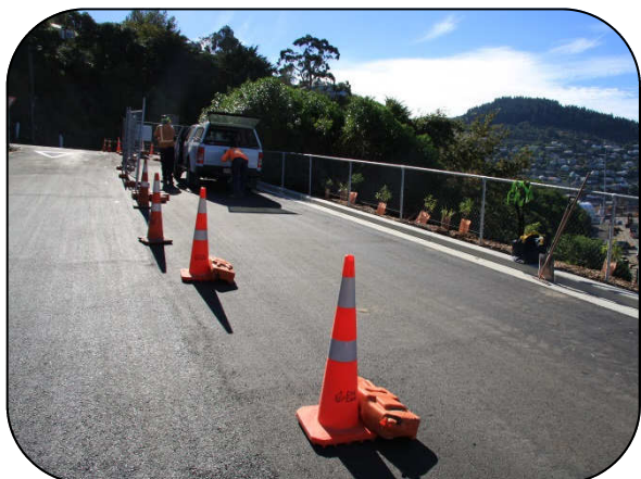
Road sealing and kerb and channel work is complete in the work area after delays caused by storm events.
