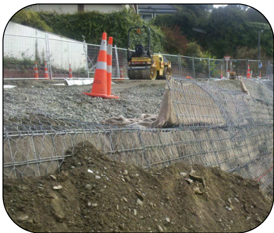
Preparation of the new reinforced soil slope. Fabric is wrapped on the front face to assist grass growth.
