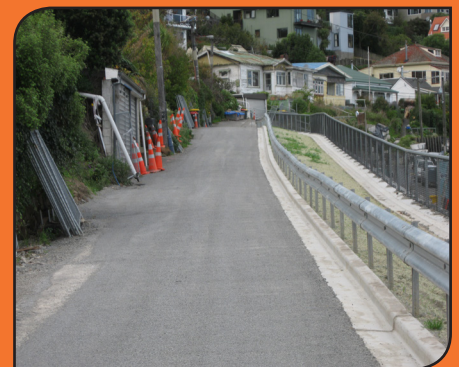
Stage 2 Sumner Road sealed.
