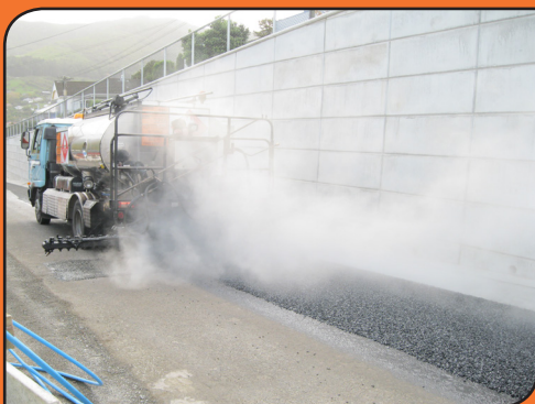
Bitumen spayer truck on Sumner Road.
