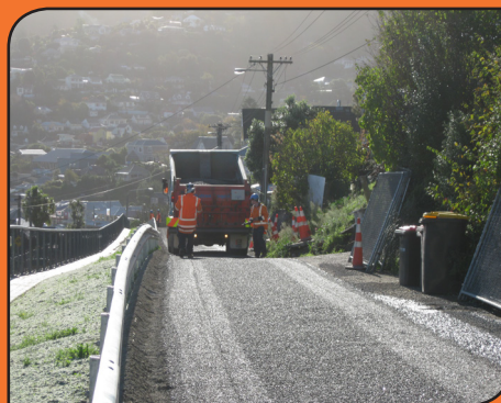
Chip seal spreader on Sumner Road.
