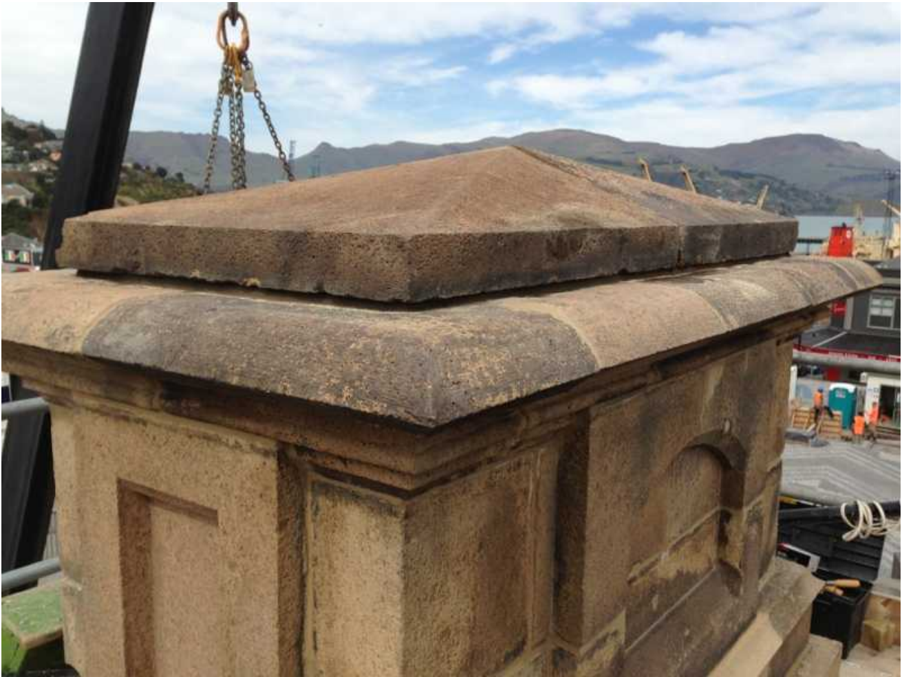
Cenotaph capping stone completed.
