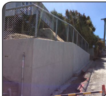
Completed retaining wall on Ticehurst Road.
