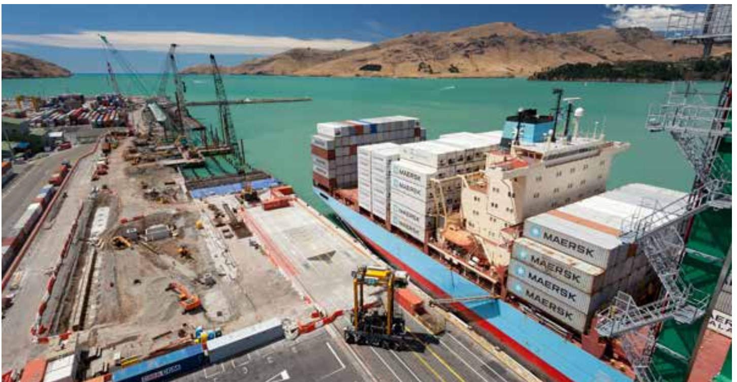
The 266 metre Lars Maersk container vessel occupying the new berth at Lyttelton Port’s Cashin Quay 2 wharf, while the Pacifica’s Spirit of Endurance is berthed beside it.
