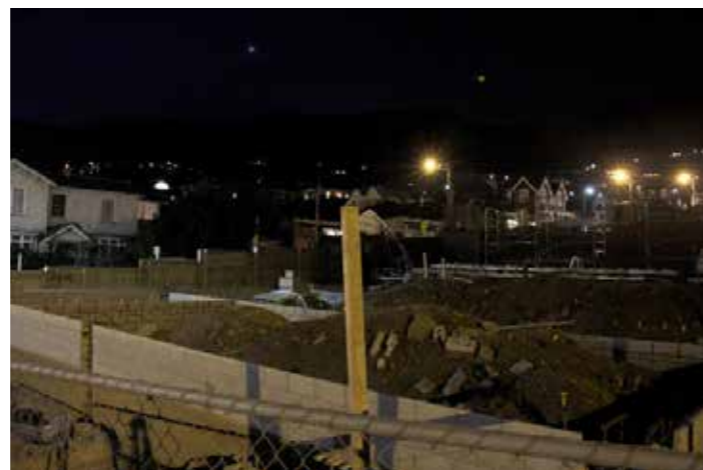
The LAF - Lyttelton Arts Factory foundations on site are well underway. Next time you're passing check out the progress for yourselves!
