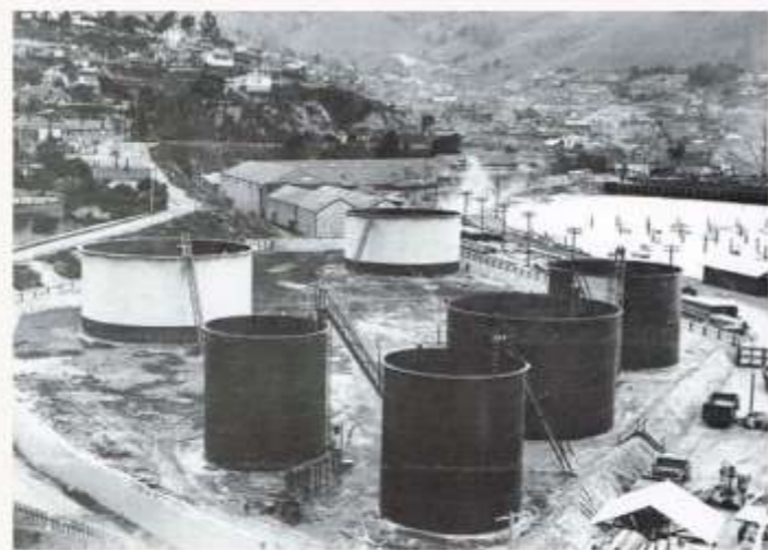
One of the first photos of the pile moorings taken in 1926. Note the stock pile of piles on the shore waiting for placing. (From Lyttelton: Port and Town - Rice 2004)
