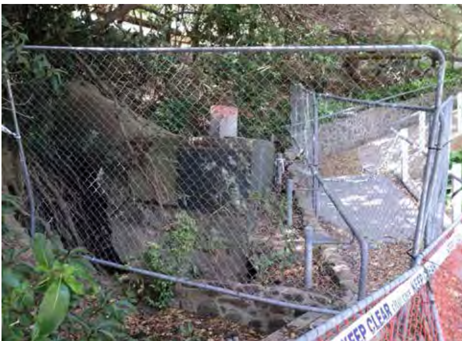
Damaged storm water pipe and subsequent hole. Closed public path in the background.
