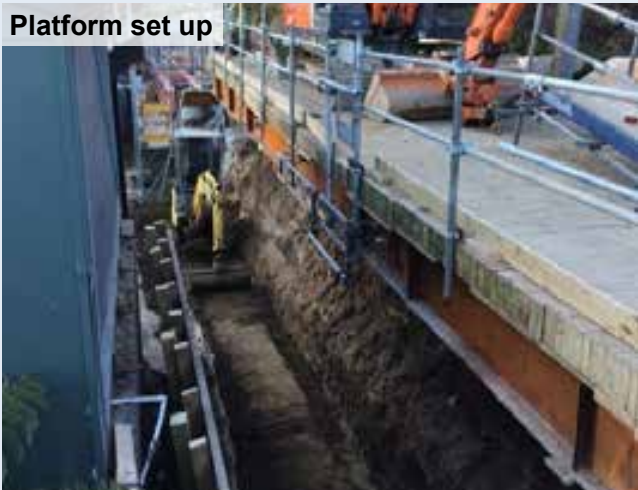
Retaining Wall installation
