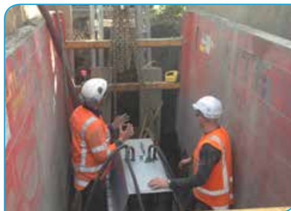
The pulling unit inside the exit trench
