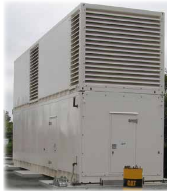
Above: One of the two 40ft, 2500 kVA generators being temporarily relocated to the Lyttelton Port Company to supply generation during the upgrade
