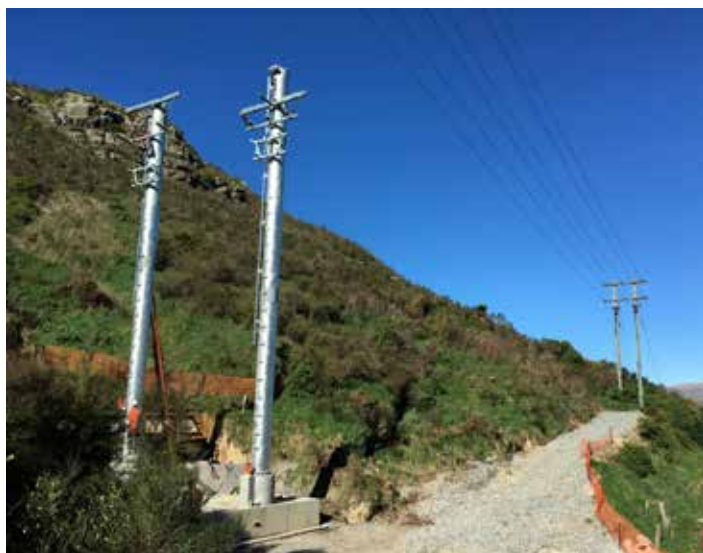
Orion New poles for 11kv line Poles
