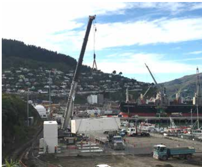
Orion Generator being lifted onto LPC
