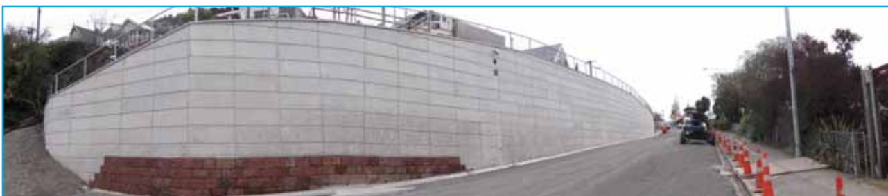
Above: Dublin Street retaining wall
