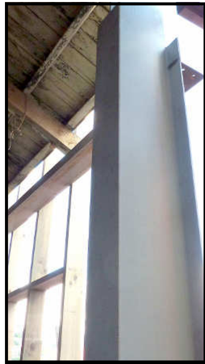
Plenty of steel for increased earthquake strengthening.
