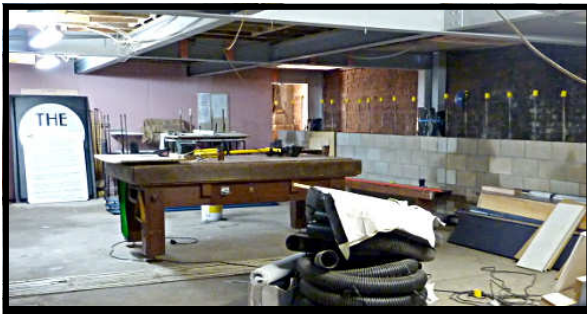
Proposed downstairs bar, shows new reinforced concrete block retaining wall to the North.
