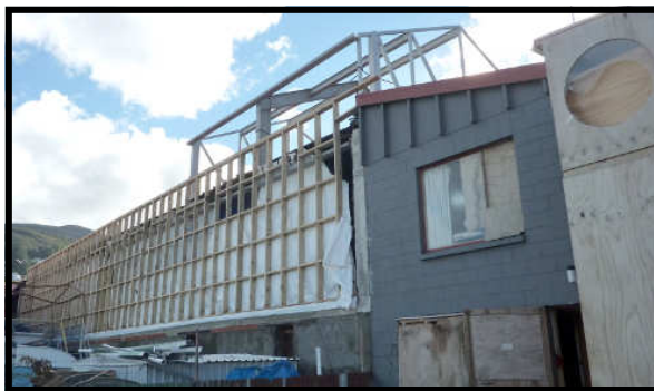
Steel framing for the new fly tower is exposed.
